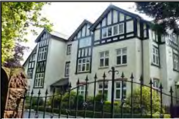
Photograph 73: Altenbrook, Harrop Road
