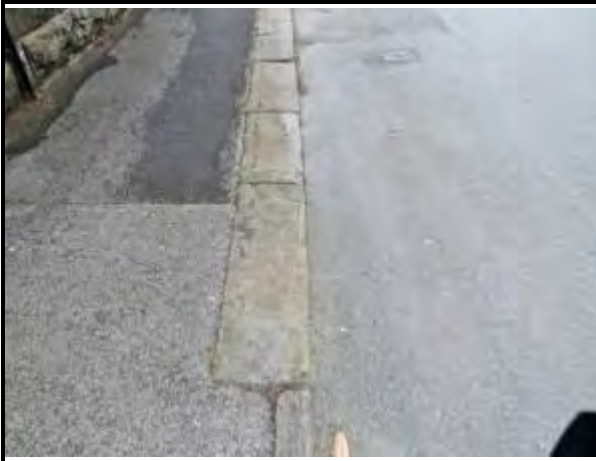
Photograph 27: Stone Curbstones (Avon Road)
