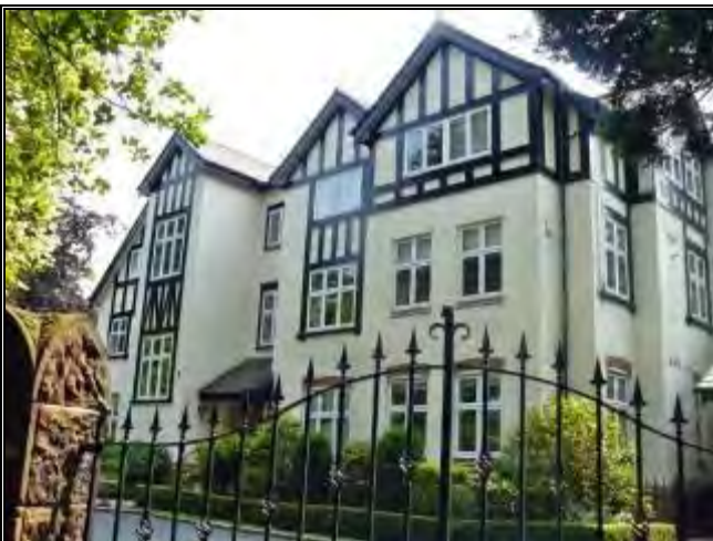
Photograph 132: Altenbrook, Harrop Road
