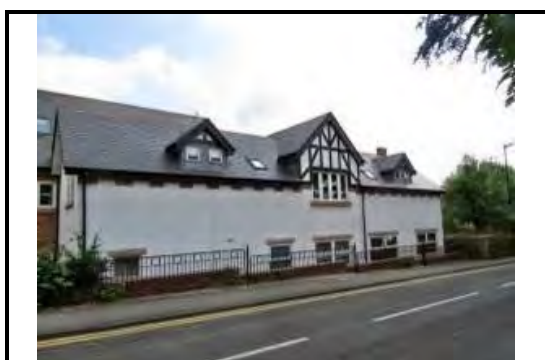
Photograph 35: Former Premises of Hale Motor Company
