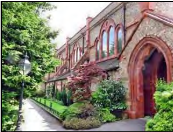
Photograph 6: St. Peter's Church North Facade
