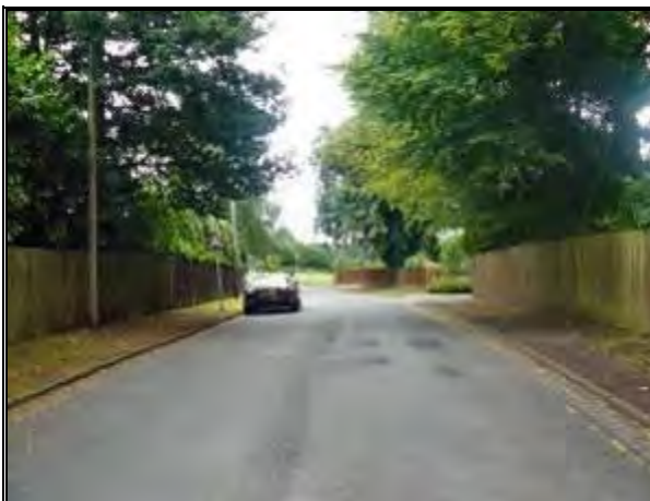
Photograph 107: View along Rappax Road
