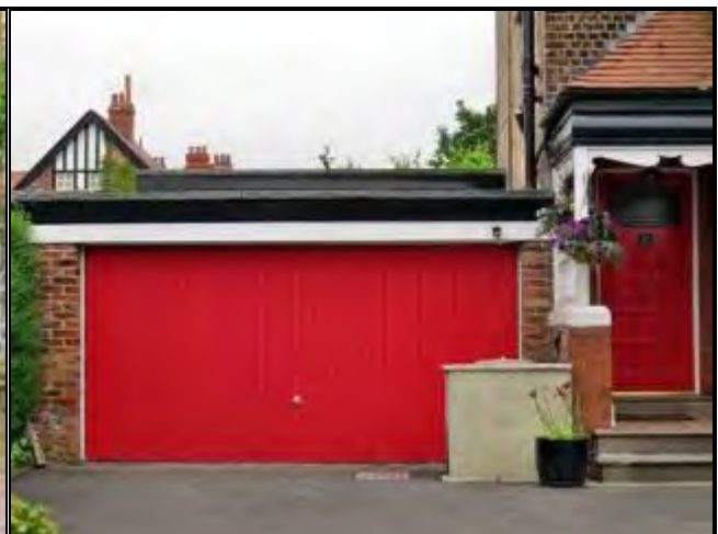
Photograph 116: Inappropriate Garage to 17 Warwick Road
