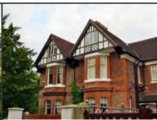
Photograph 21: 251 & 253 Ashley Road with Jettied Gable and Pantile Roof
