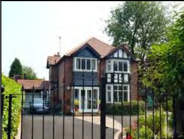
Photograph 111: UPVC Windows and door surround to 8 Harrop Road
