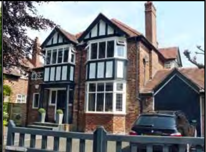
Photograph 112: UPVC Windows to number 3 Bower Road
