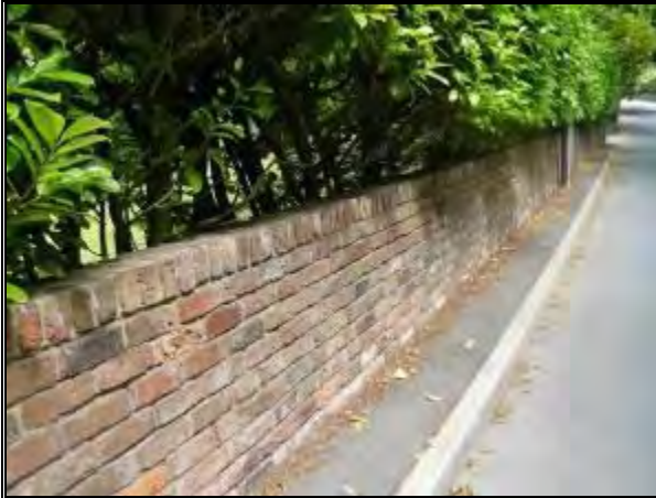
Photograph 105: Modern Brick Wall, Bankhall Lane
